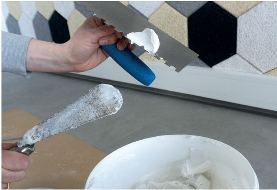
1: Add a small amount of FibroTech assembly adhesive on a putty knife or a similar tool.
